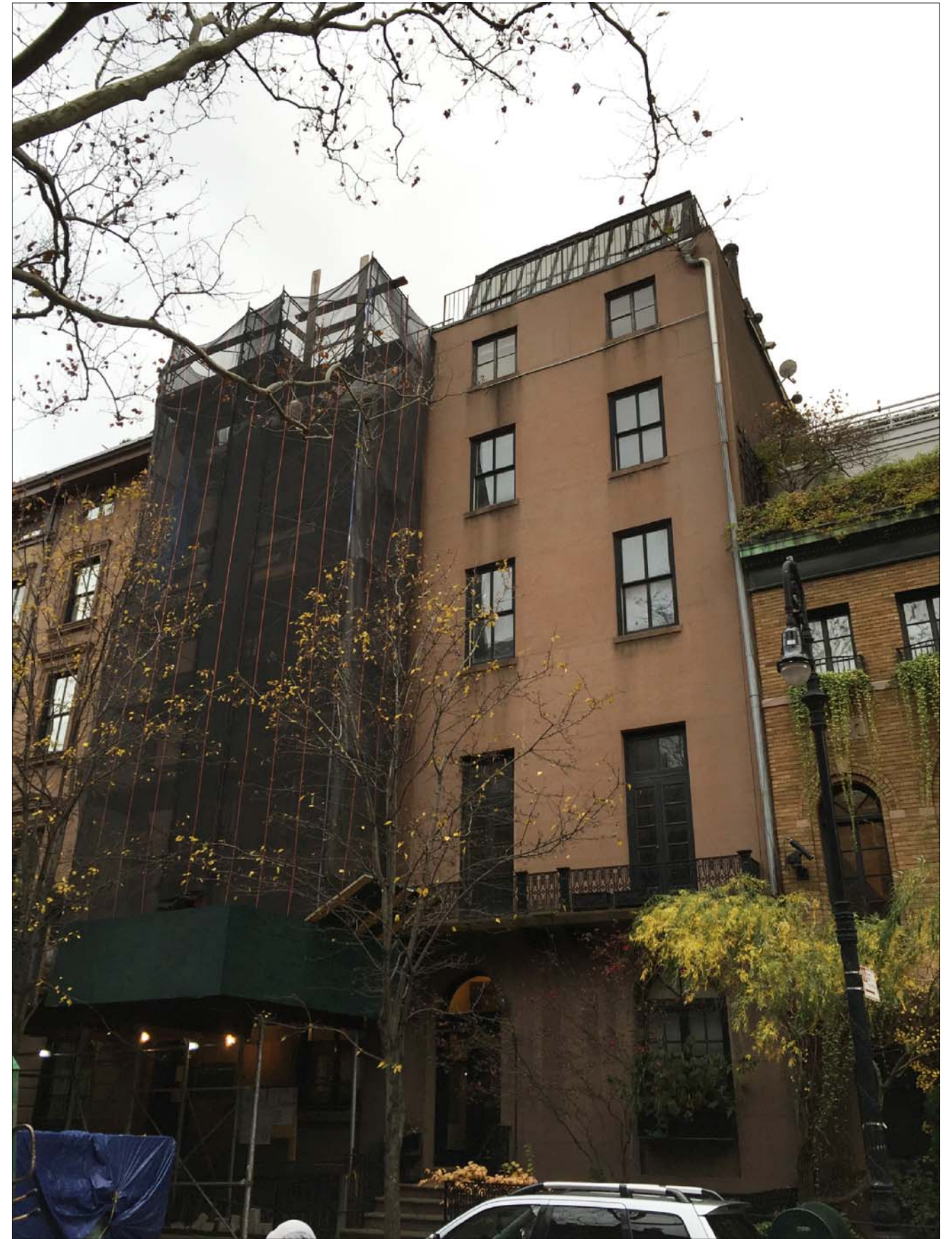
Existing Street Facade - No. 38
