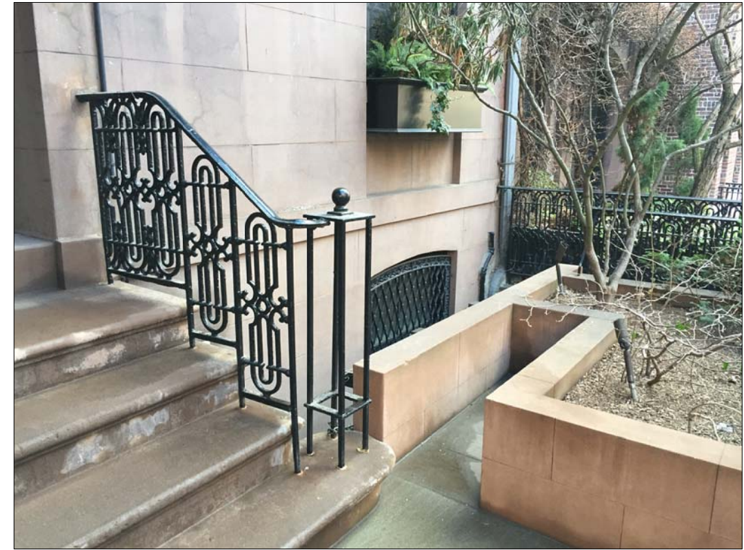
EXISTING RAILING & NEWEL POST AT NO. 38
