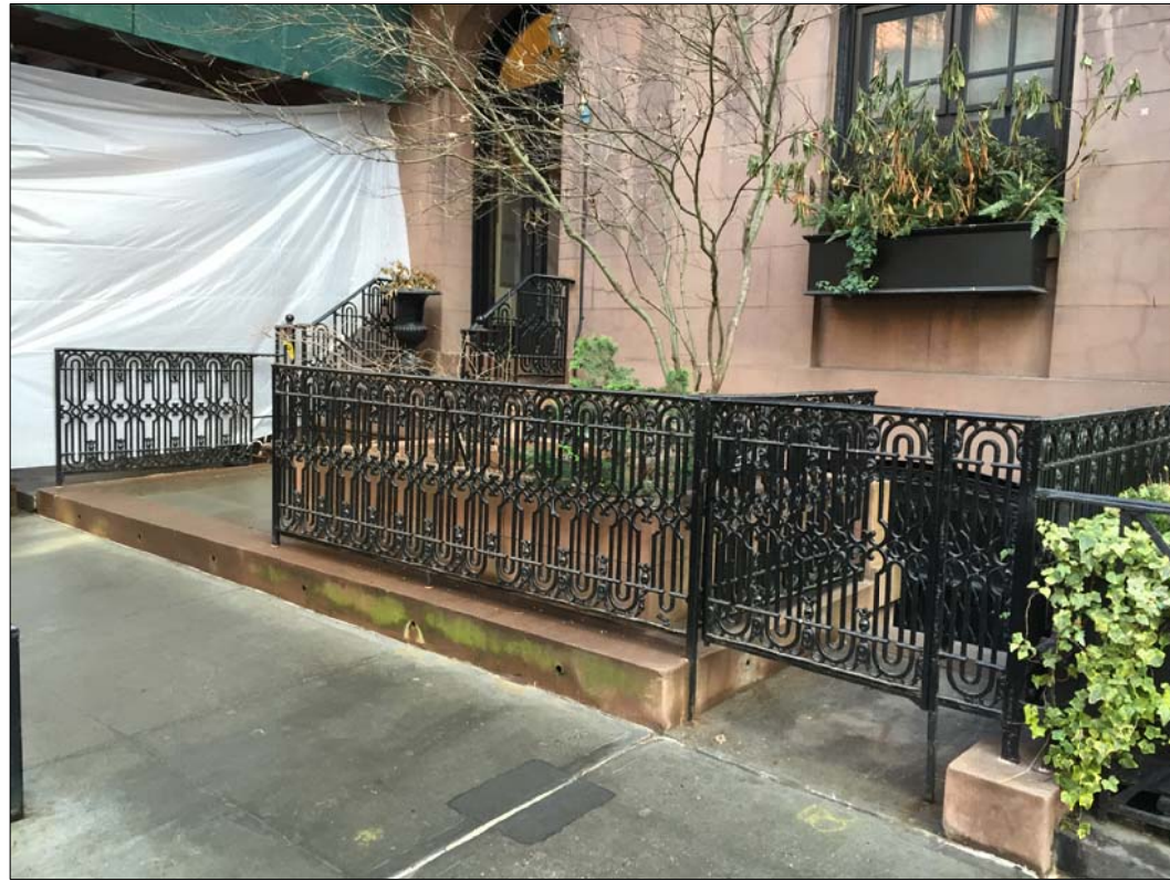
EXISTING FENCE AT NO. 38
