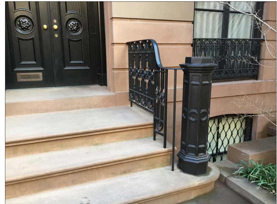
EXISTING HISTORIC RAILING AND NEWEL POST AT NO. 34
